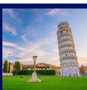
Leaning Tower of Pisa
